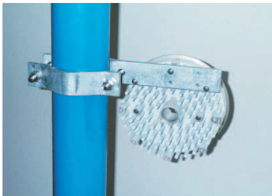
Figure 21: Indirect-mount bracket on pole
